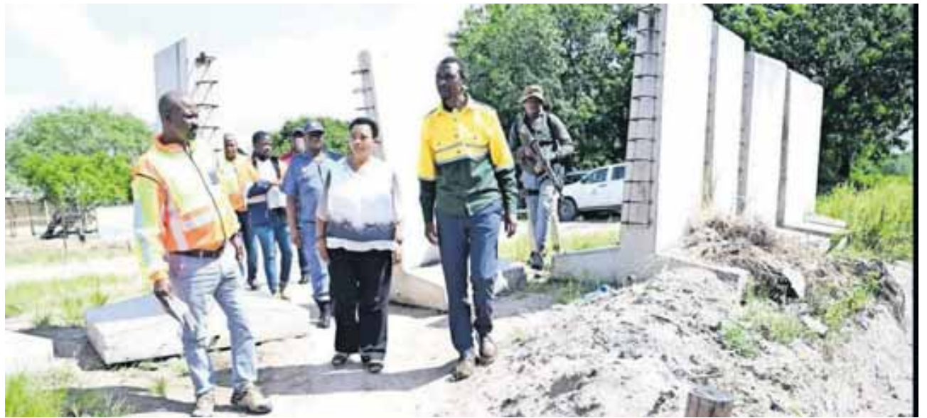
■ The KZN Premier Nomusa Dube-Ncube inspects the concrete barrier wall between the South African and Mozambique border. The KZN government say they are focused on fighting crime in the area, especially the movement of illicit goods and the theft of vehicles from South Africa to Mozambique.
